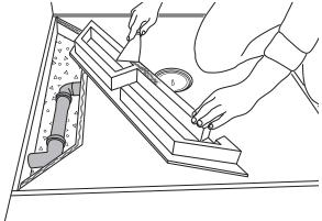
7) Then apply tile adhesive to the underside of the pipe duct element.
